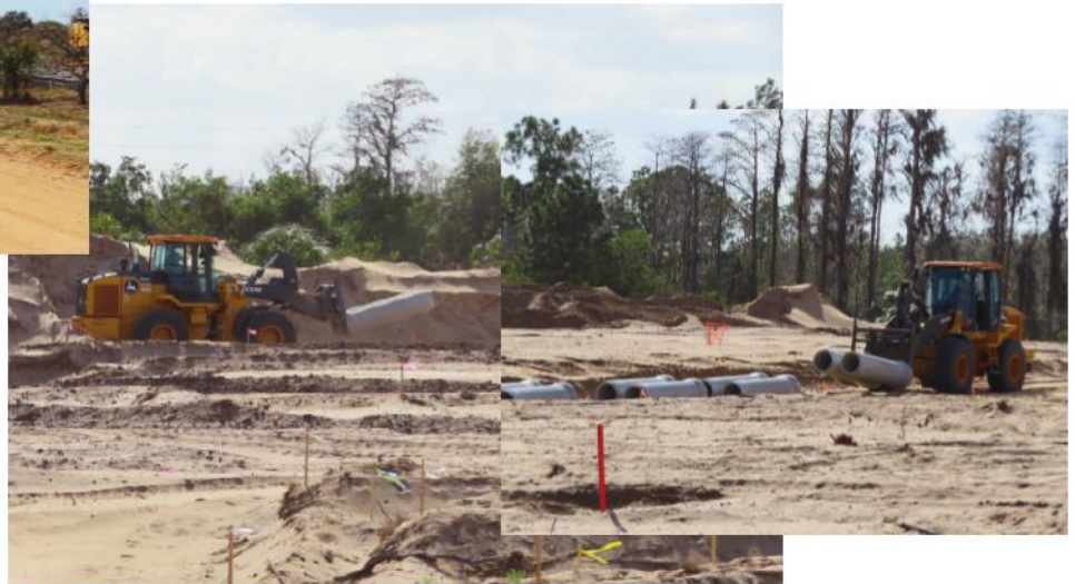
The first photo in the series shows the drainage pipes being taken off of the “delivery” truck. They are then transported down the road that leads to the church building and then placed with the others to be installed the first part of next week.
