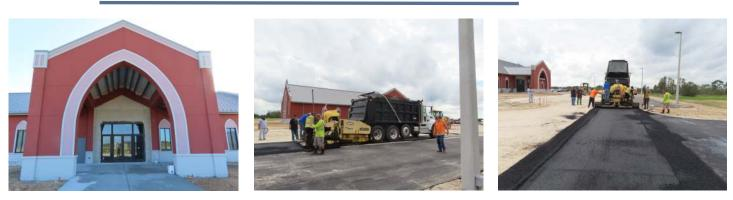
The front door has been installed, the ceilings are almost complete, interior light fixtures and floor tiles are in various stages of completion, and the air conditioning was turned on to circulate the air for priming and painting. Outside we see the blacktopping of the parking lot and roadway. For all the construction photos, starting with the January 19 clearing of the land, please go to our website at: Construction Update - St. Faustina Catholic Church - Clermont (stfaustina.org)
